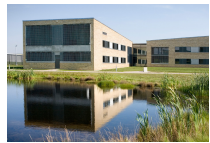
Denmark Enner Mark Prison
