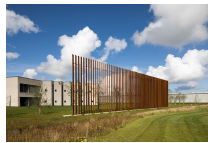
Denmark Storstrøm Prison
